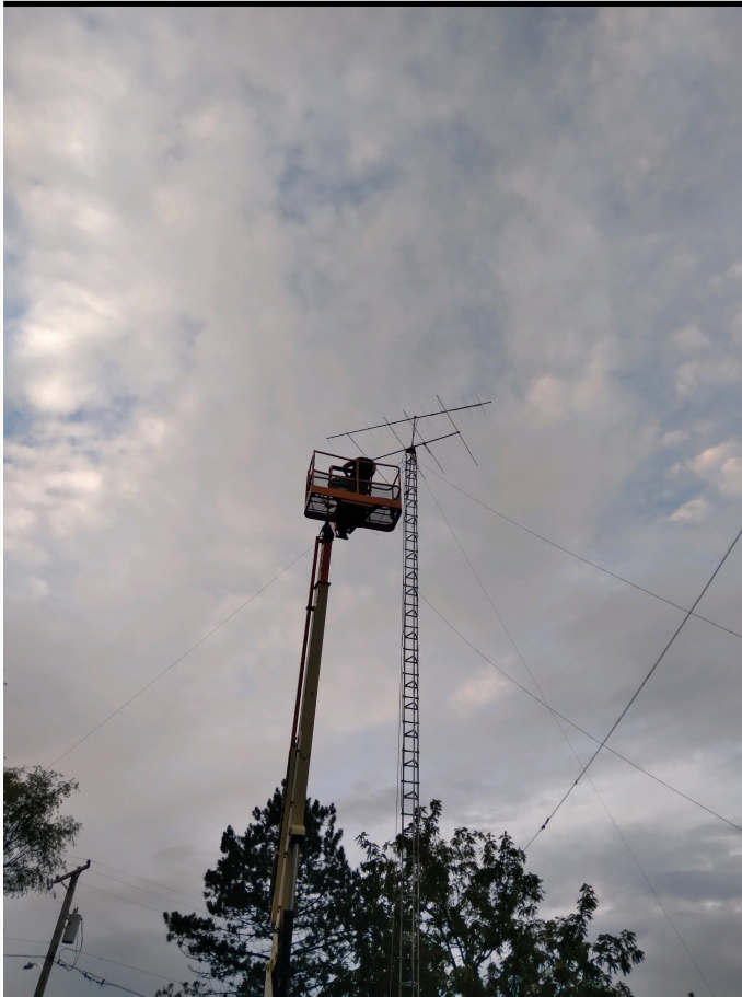
Recent work at QTH of Mike-W8CJJ in dismantling of his tower/antenna farm
