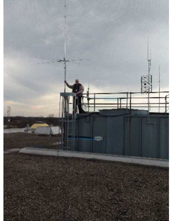
WD8LEI with vertical installed
