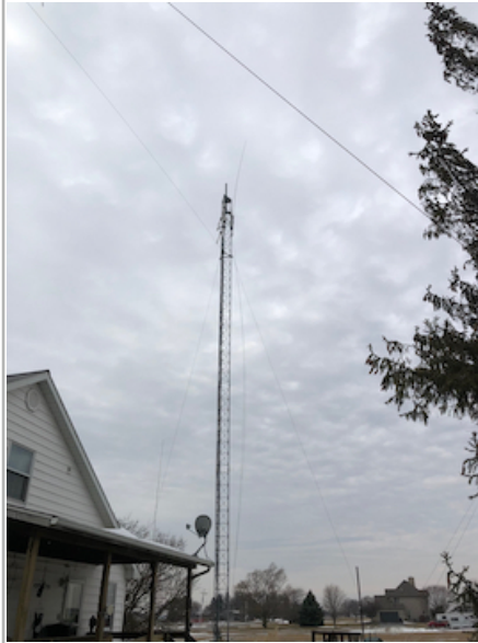
Recently Erected Rohn Tower
