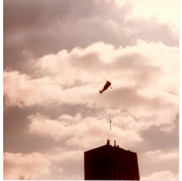
Tower is put in place
