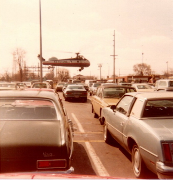
Helicopter prepares to lift tower
