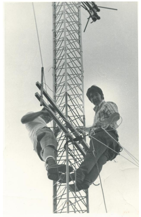
Installing WCARC repeater antennas—guess who?
