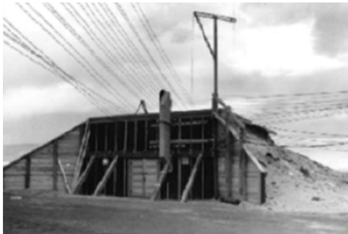
Trinity Site - Main Bunker
