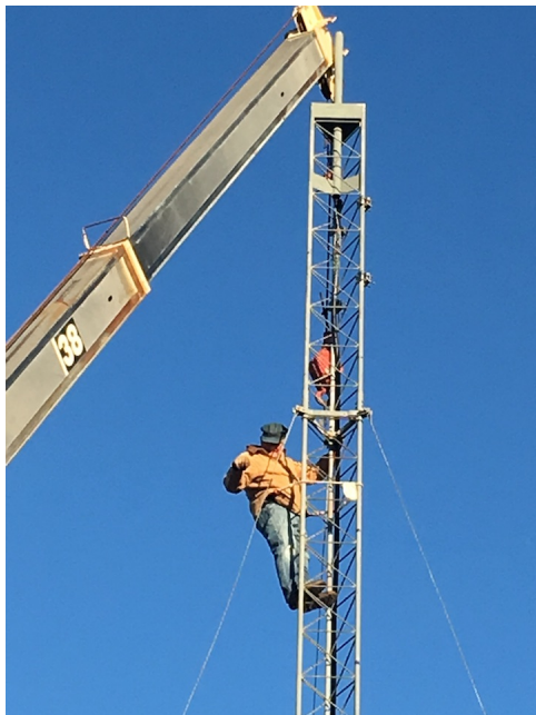
crane hook released
