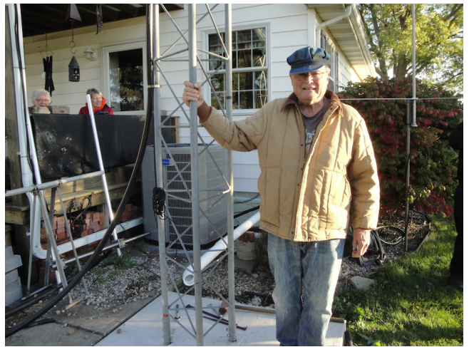
WB8NQW after tower is secured
