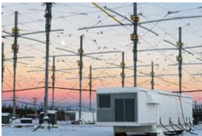
A section of the extensive HAARP antenna array and one of the transmitter shelters. [Photo courtesy of KL4IU]
